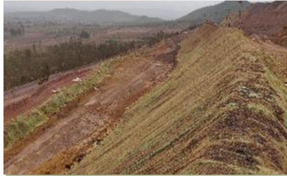
Spreading of Geo Coirmats on the dumps in order to retain fertility and vegetation
