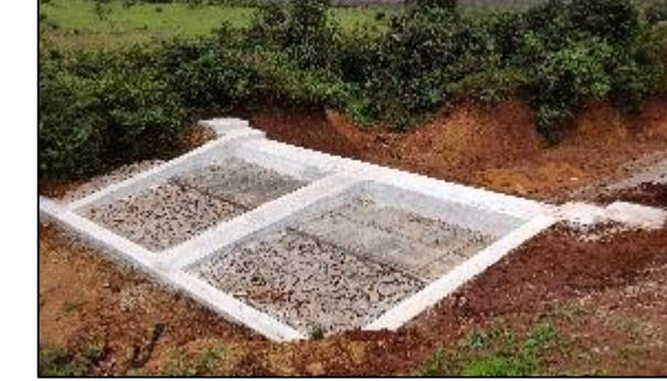
Newly constructed Checkdams on natural streams in forest area has a capacity to store 4800 m 3 of rainwater
