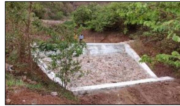
Newly constructed Checkdams on natural streams in forest area has a capacity to store 4800 m 3 of rainwater
