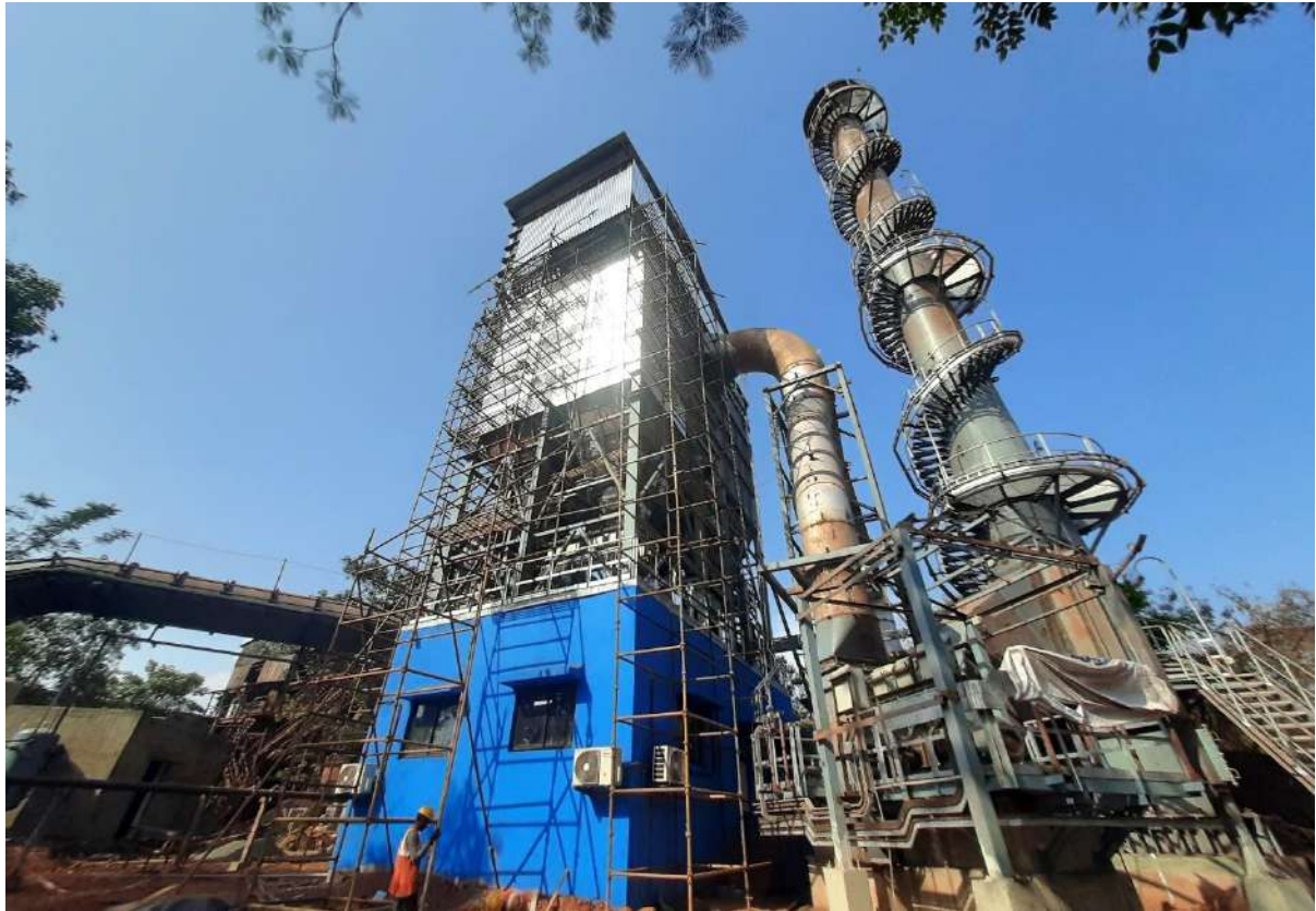
New Baghouse installed for Blast Furnace-1
