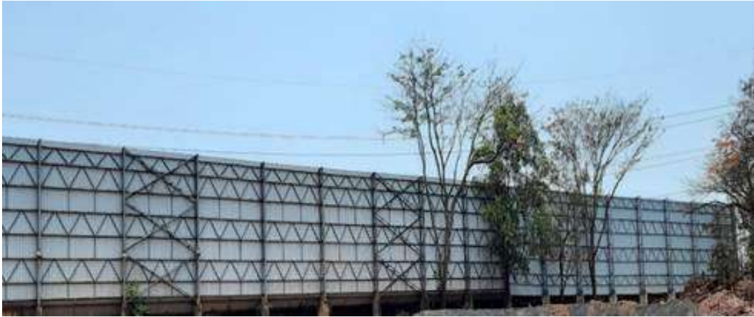
Windshield installed towards Amona village side
